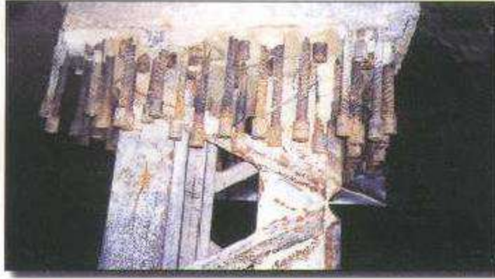
Top – Down Construction
