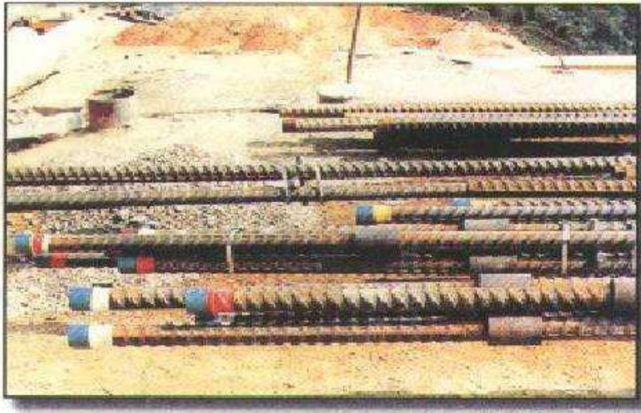
Micro piles & Soil Nails
